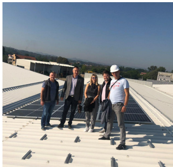
Figure 24. Solar panels of IMACO Systemtechnik
